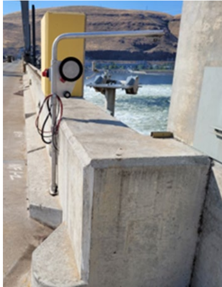
Figure 2: Image of crab hauler extending beyond the safety ledge.
